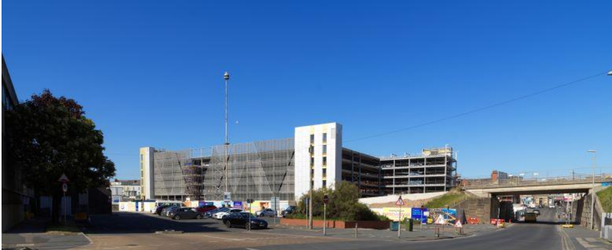
New Multi Storey Car park under construction
