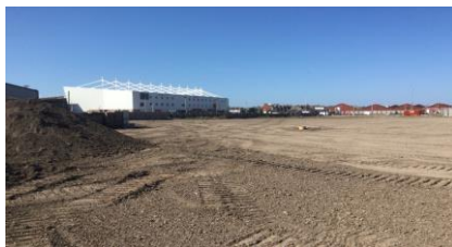
Cleared site behind the football club North Stand
